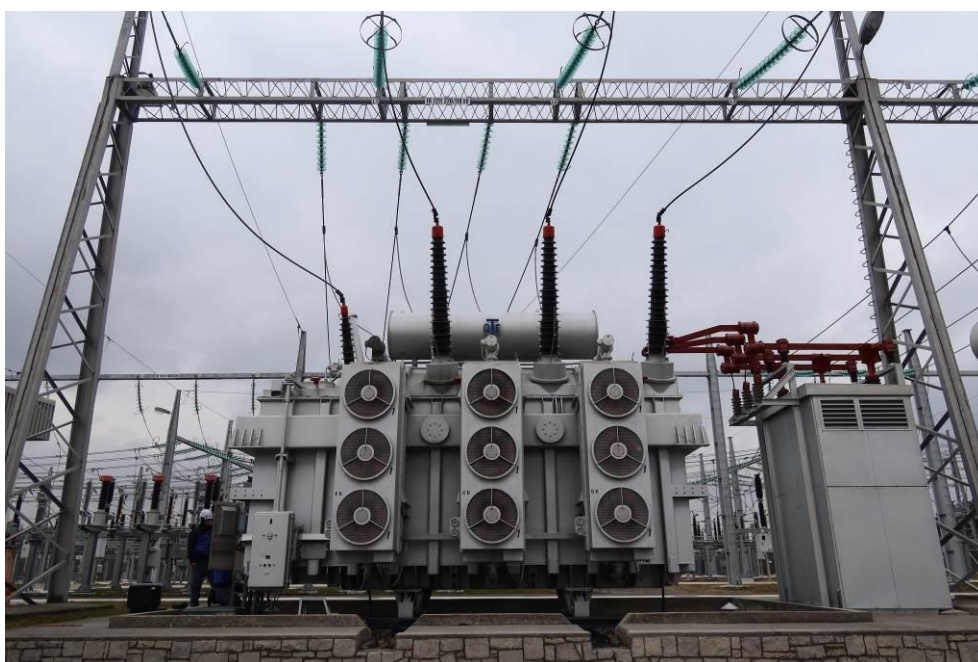
Picture 15: power transformer 220/110 kV - T212
