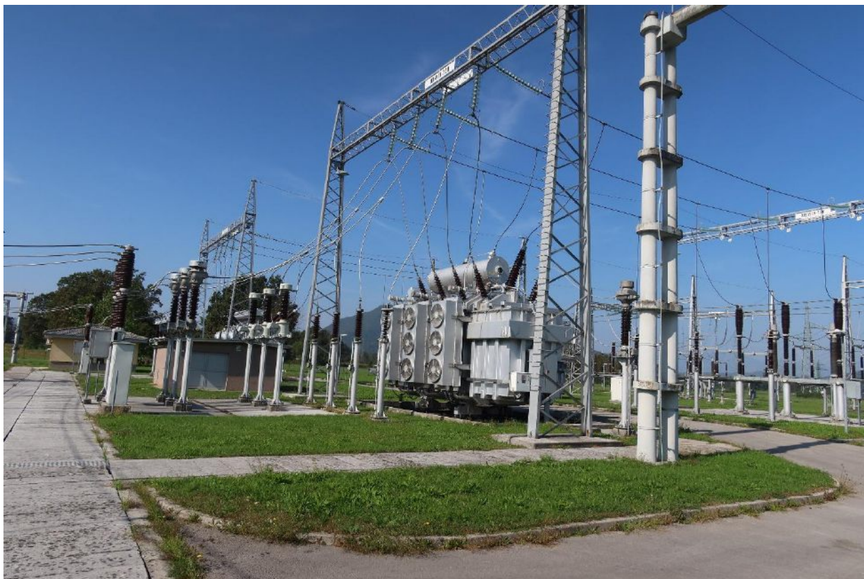
Picture 11: power transformer 220/110 kV - T211
