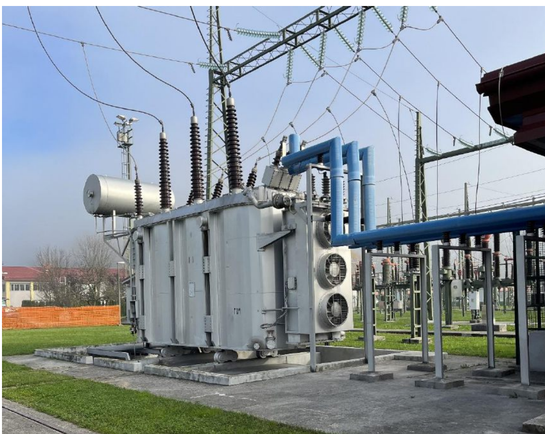
Picture 3: power transformer 220/110 kV - T211
