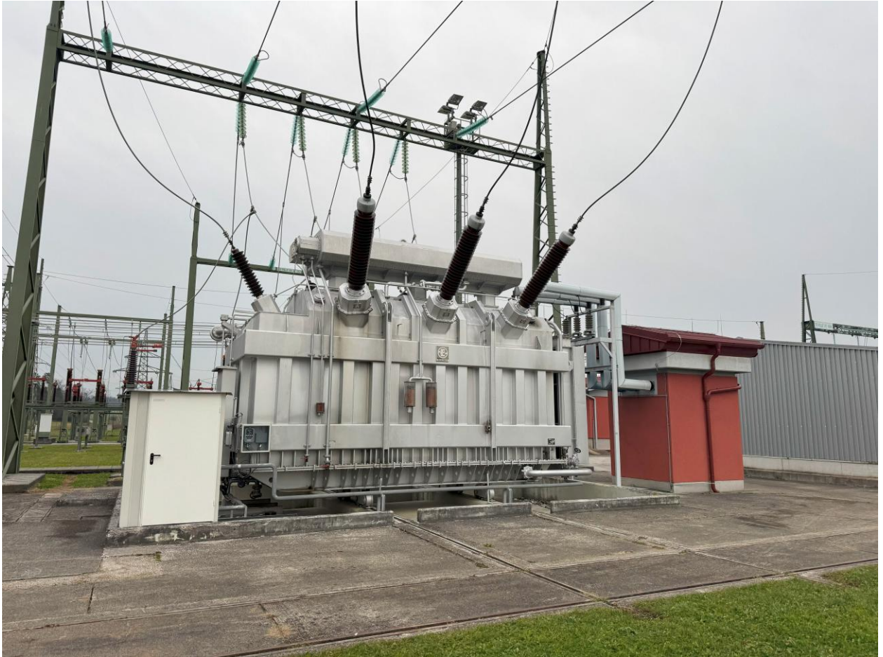
Picture 5: power transformer 220/110 kV - T212
